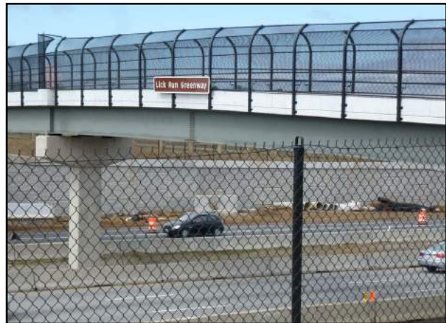
When Valley View interchange over I-581 was rebuilt, a separate bridge was provided for Lick Run Greenway.
